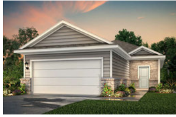
The Enclave at Sonterra Jarrell
